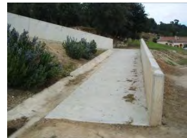
Detall rampa sense passamans (Comptals)
