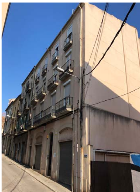
Façana carrer Hospital, 12-14
