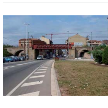
Tram principal del pont
