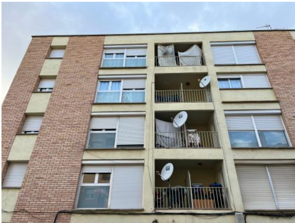
detall façana principal
